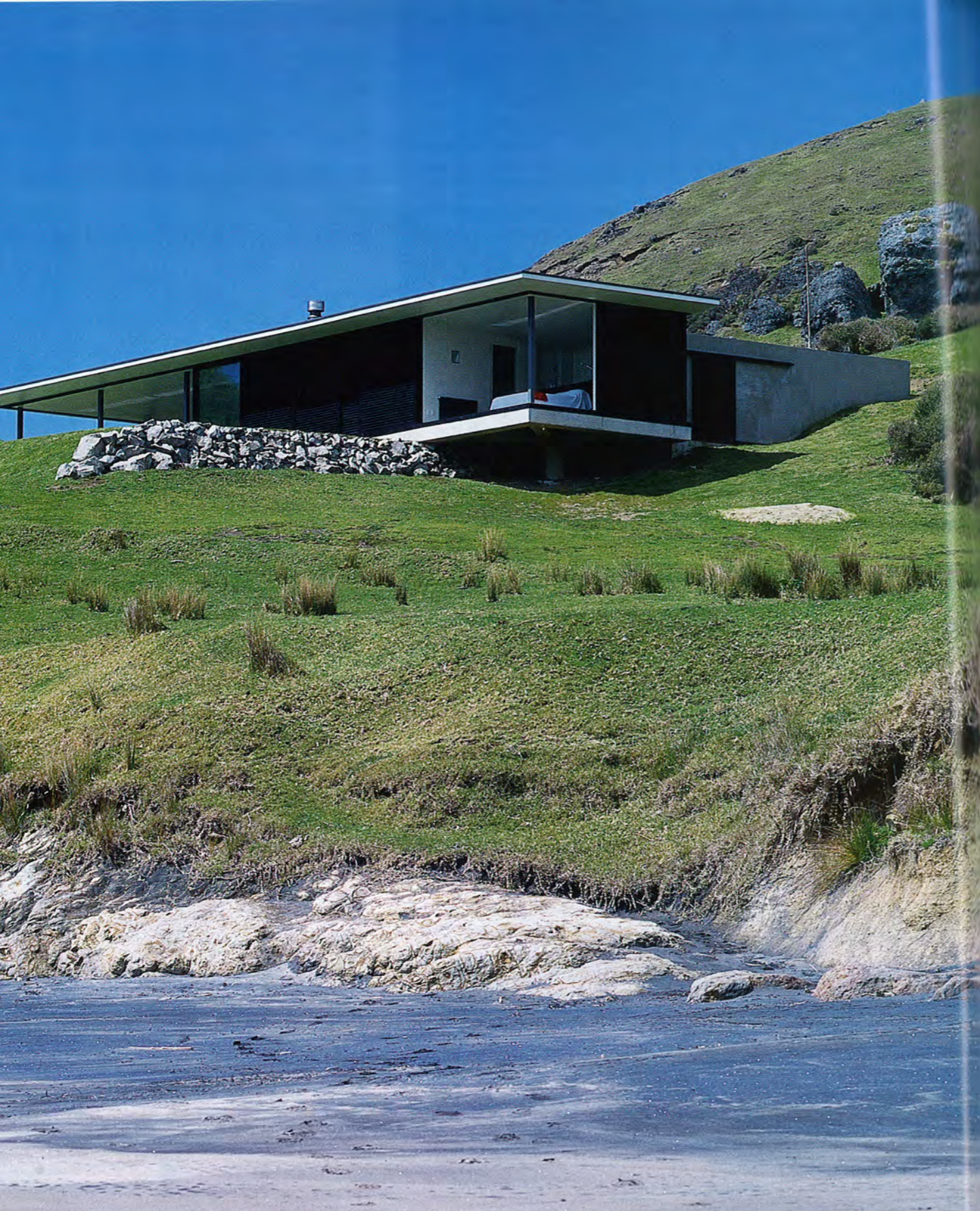
The house is sited along a remote and craggy cove, just where a steep slope levels off into flat, grassy terrain extending out to the surf (above and opposite). The master bedroom, at one corner of the building, cantilevers off the ground. The structure also sits on a low wall of stones, collected from the site (above).
